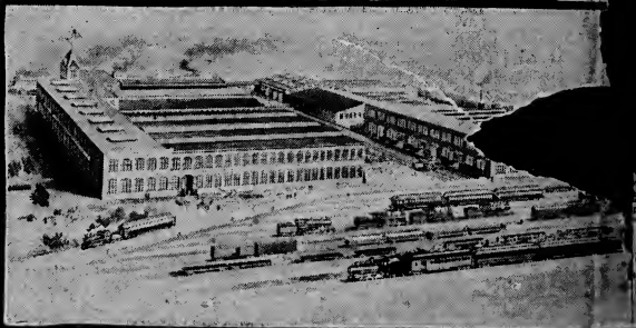
THE HICKS MAIN PLANT
